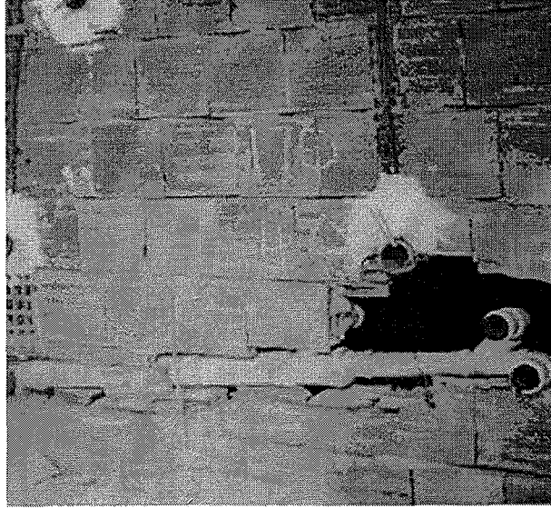
Figure 1: Material waste due to imperfect planning of construction.
