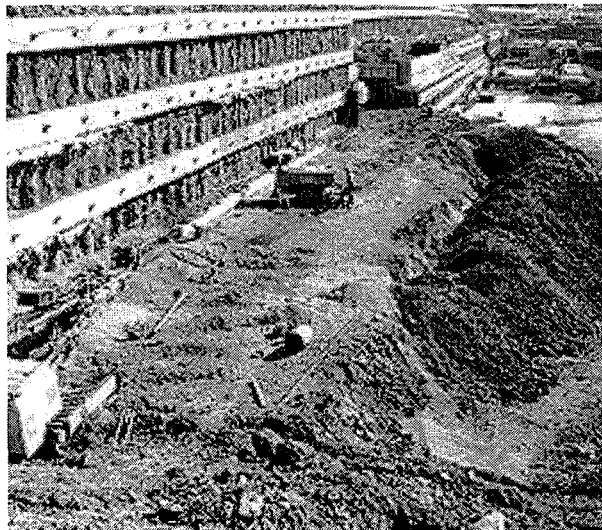
Figure 2: Material waste resulting from overordering due to mistake in quantity survey.
