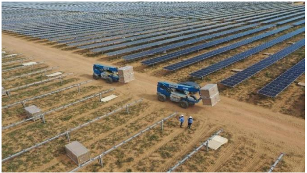
Photovoltaic Energy Construction
