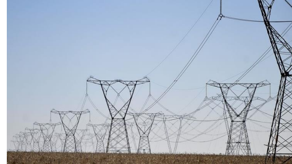
Power Transmission Lines Construction
