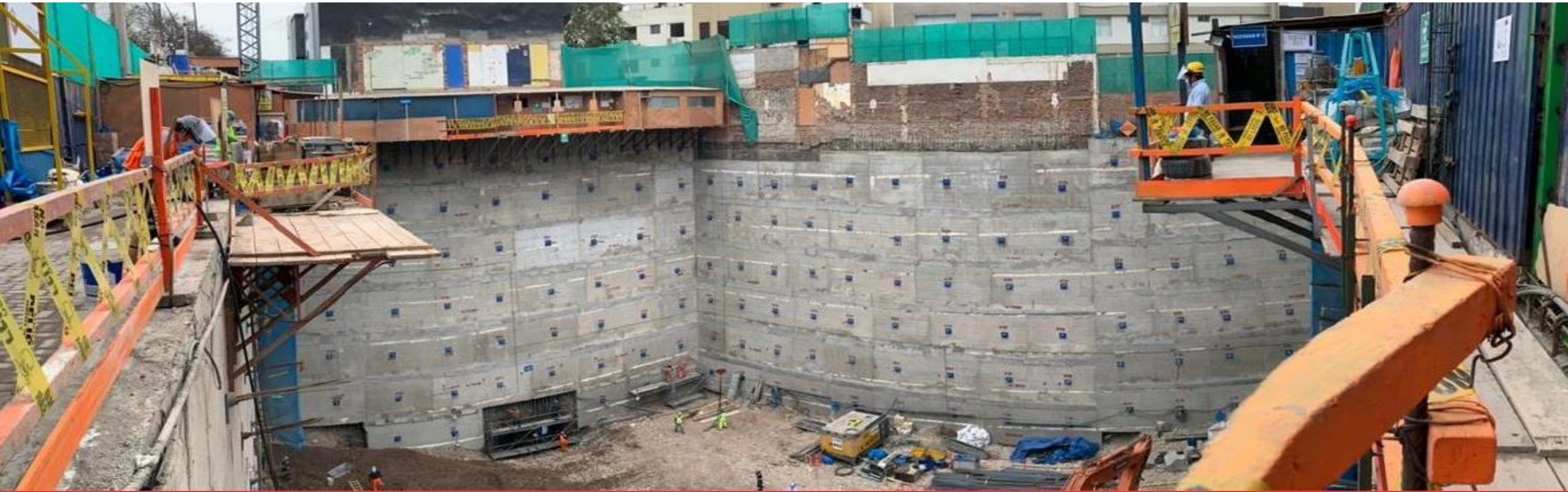
Figure 2. Panoramic view of the building of the anchored wall
