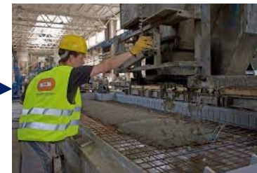
Concrete casting (m3)
