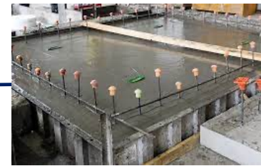
Concrete curing (m4)
