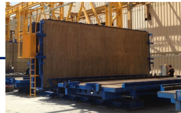
Formwork dismantling (m5)
