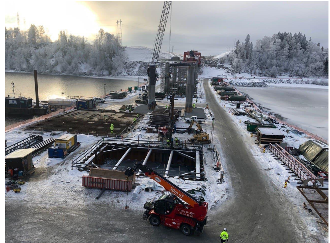
Figure 1. Minnevika Bridge Project
