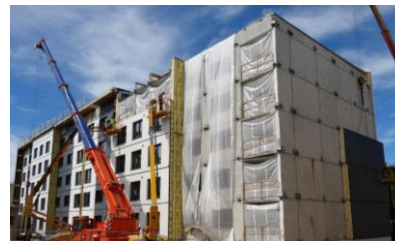
Installation on site
