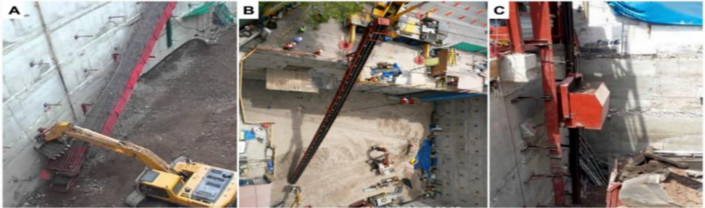
1) Removal by conveyor belt anchored in walls
