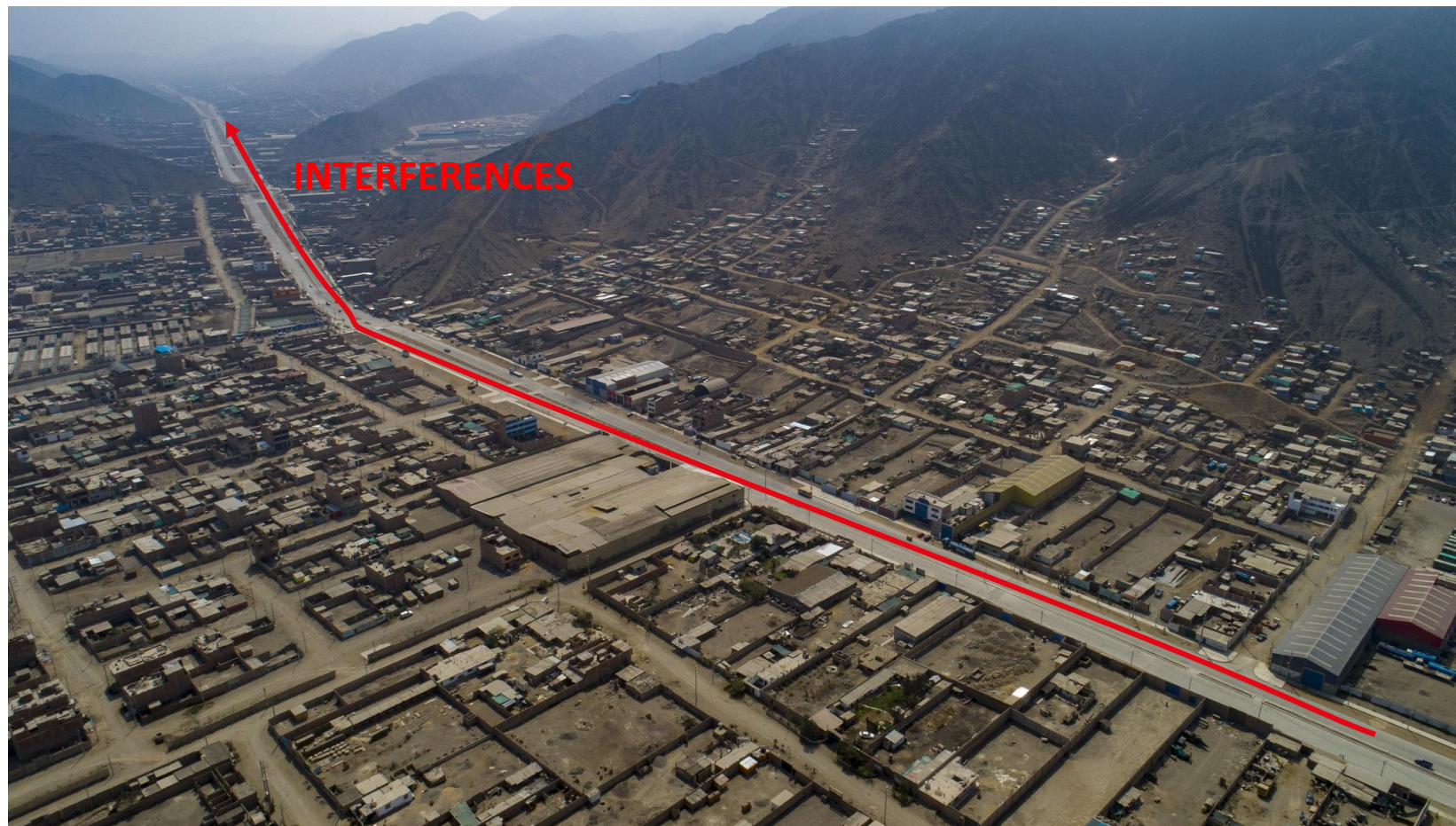
Figure 4. Case study project
