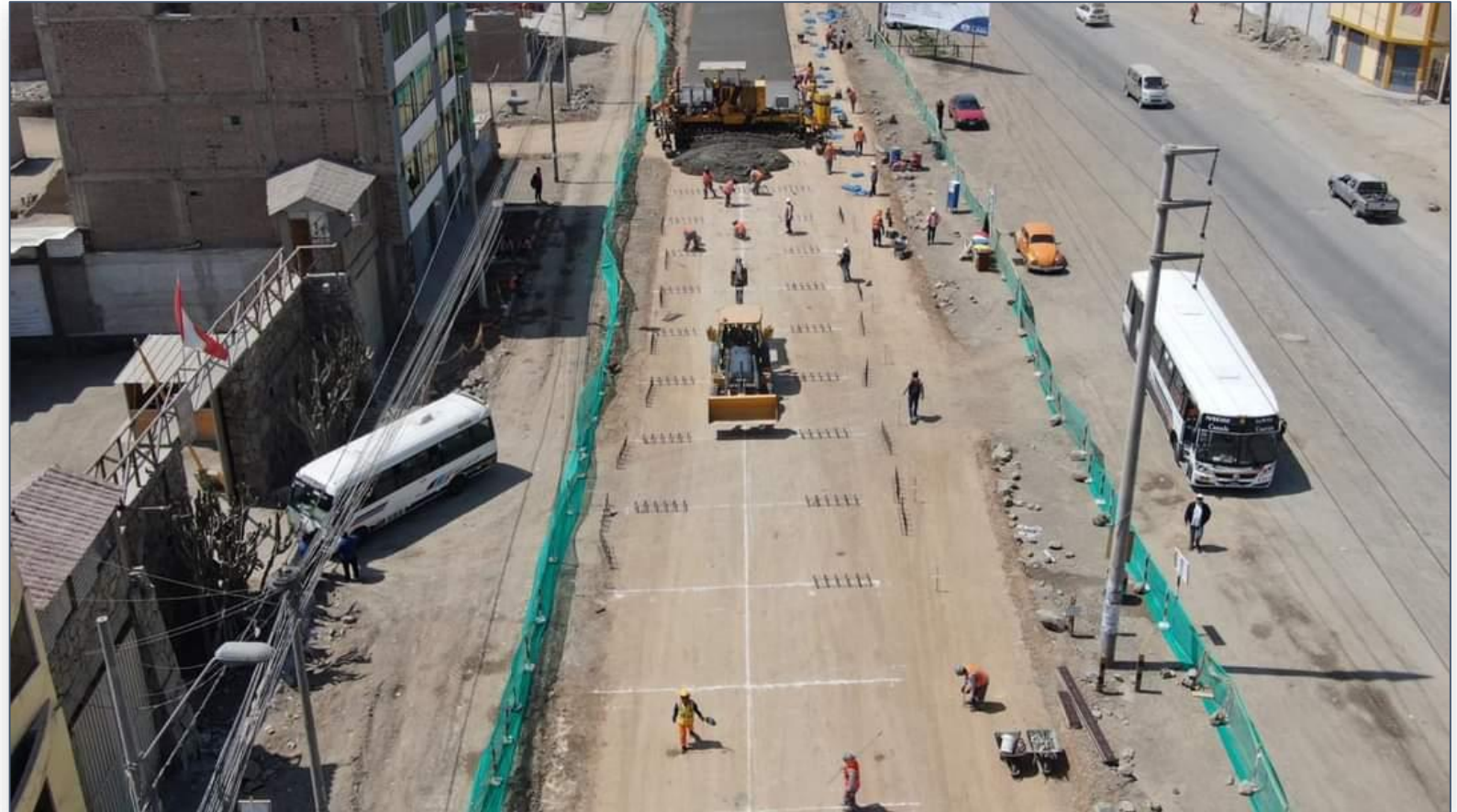
Figure 2. Road construction site
